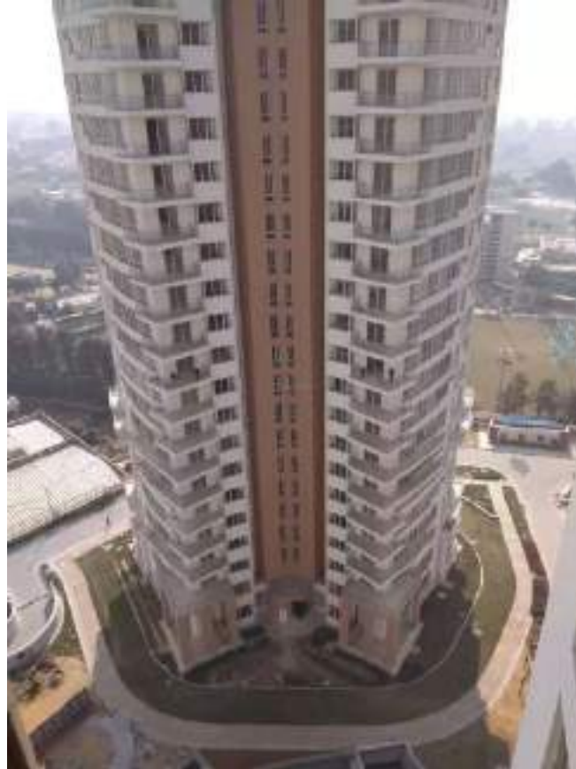
Presedia 228 flats, all 5 towers handed over
